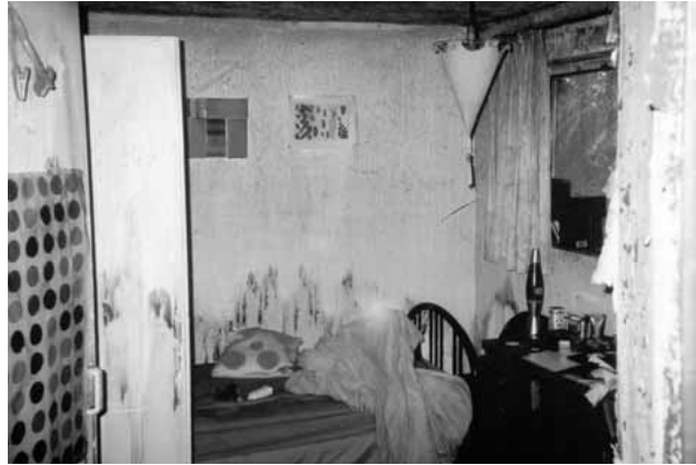
Fire Damage due to misuse of fire doors
